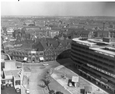
The Tesco store at the bottom of the new six-tier "Multi-Dek" car park at Lee Circle, Leicester
